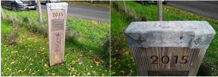
**Finding:** Lead flashing has been used to form a cap on the **Action:** Refer to the supplier for a toxicology assessment top of the sign
