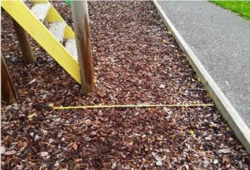
**Finding:** The edging forms a hard object within the impact area of the equipment in contravention of the requirements of BS EN 1176 Part 1
